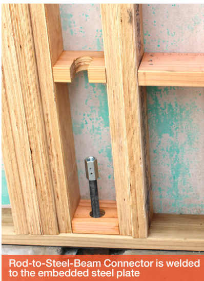
The ATS threaded rods are ready for the second floor to be attached above
