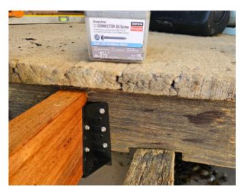
The FREP hangers and connectors ensured robust load transfer and long-term durability in a high-moisture environment.
