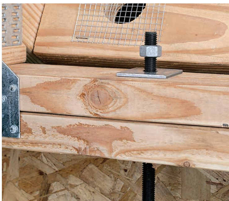
Rod system with no take-up device installed.
