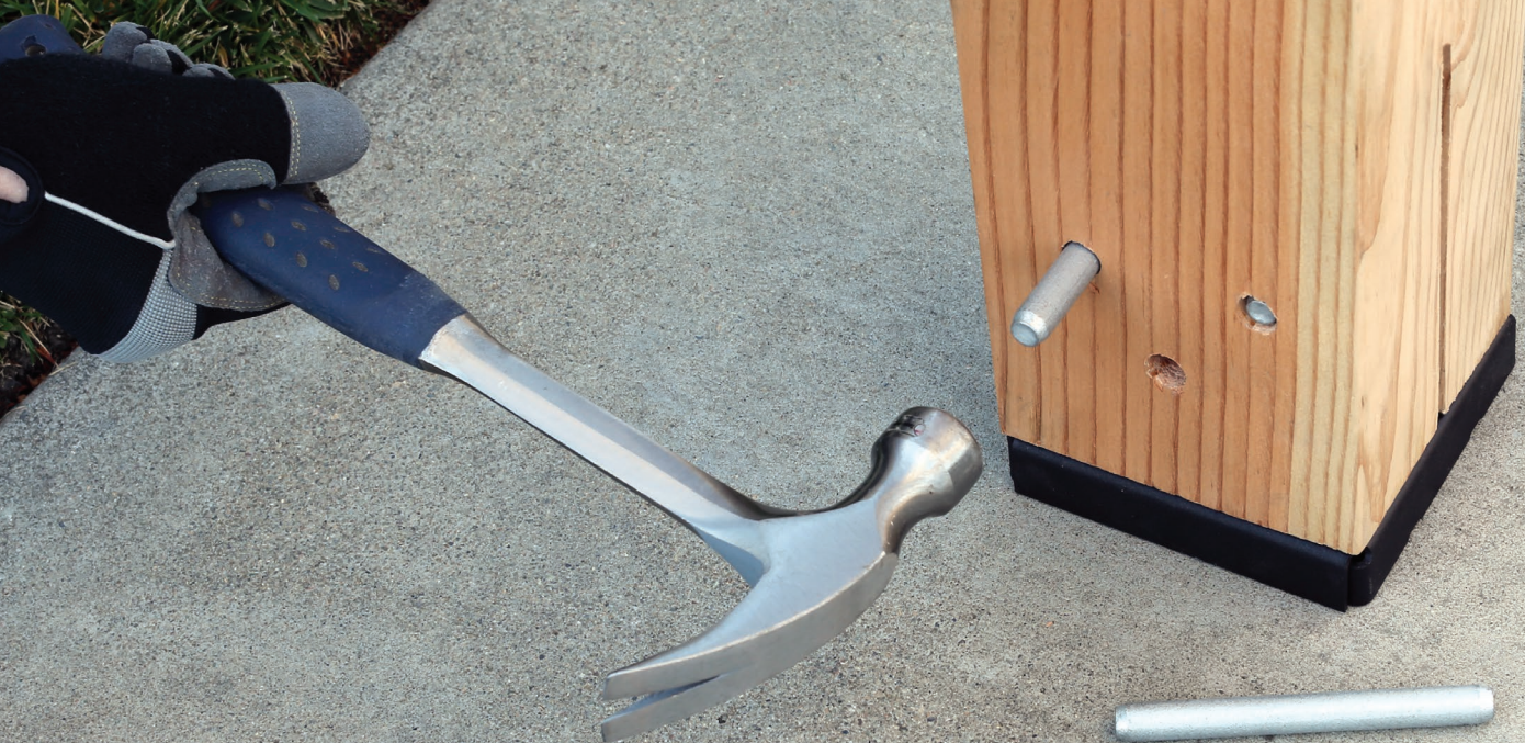
Typical CPT installation (ZMAX® 140 mm version shown)
