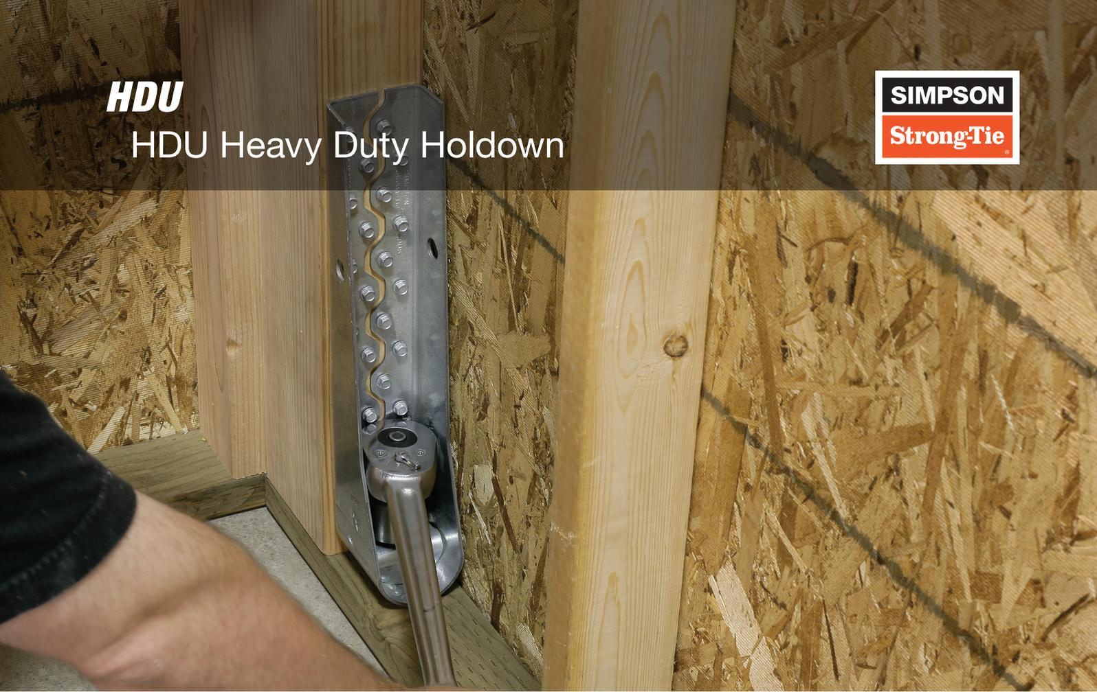
Designed for use in shearwalls, CLT wall panels, braced-wall panels, other lateral applications in wood construction.
