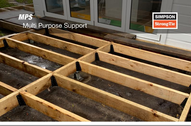
To suit bottom of bearer or joist heights from 90mm to 150mm
