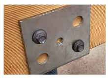
4. When fixing 65mm - 100mm wide timber to MPS use 6.4mm x 76mm SDS Heavy Duty Connector Screws.
