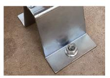
3. Fixing MPS To Concrete: 2 x 10mm x 60mm THD Titen HD Screw Anchor (THD10060MG).
