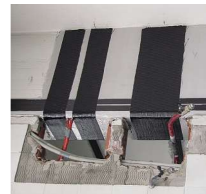
4 Beam with S&P C-Sheet 640 (Shear force)
