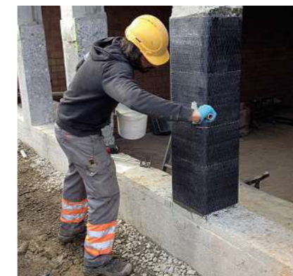
5 Column with S&P C-Sheet 240 (Normal force)
