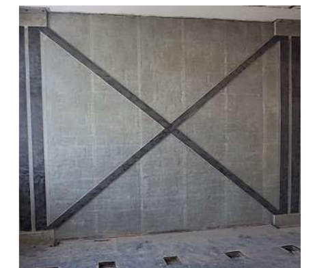
6 Strengthening of masonry with S&P G-Sheet (Seismic enhancement)
