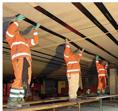
1 Surface applied S&P C-Laminate (Bending)
