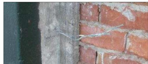
(d) Concrete shear key and wire tie connection to the boundary column
