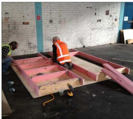
(a) Plywood backing frame being constructed
