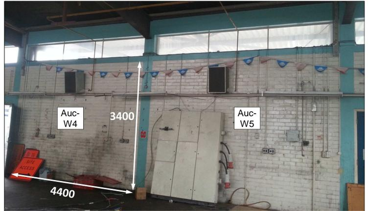
(c) Interior of west wall prior to testing with test walls labelled and dimensions (in mm) shown
