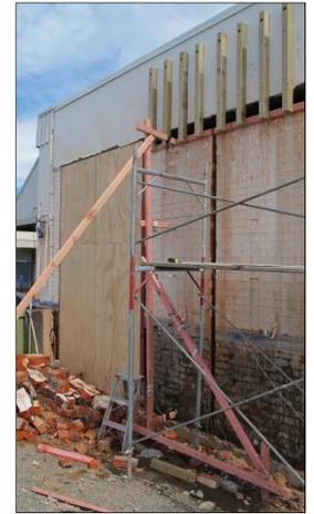
(c) Lateral timber restraint anchored to the RC beam above Has-W3 and Has-W4
