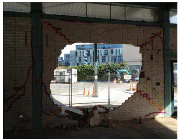
(d) Partial wall collapse post-loading on the loading side of Auc-W5
