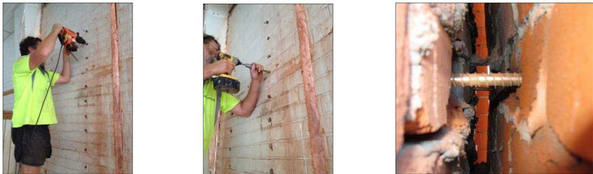
(a) Pre-drilling cavity tie holes (b) Installing mechanical ties (c) Mechanical tie spanning cavity
