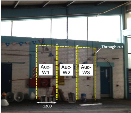
(b) Interior of north wall prior to testing with test walls labelled and dimensions (in mm) shown
