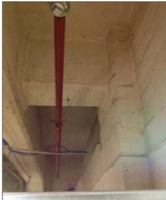
(e) Instrumented side of Wel-W2 above the suspended ceiling level showing RC beam resting on brick pier
