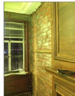
(m) Instrumented side of Wel-W6 after gypsum board removal and vertical saw cuts made
