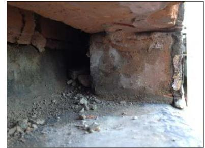
(c) Exterior cavity wall with brick removed exposing the lead damp-proof course and air gap cavity
