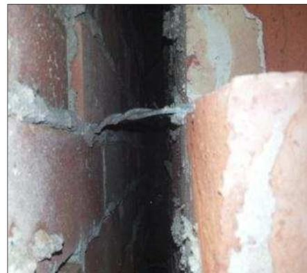
(b) Twisted wire cavity ties in mortar joints
