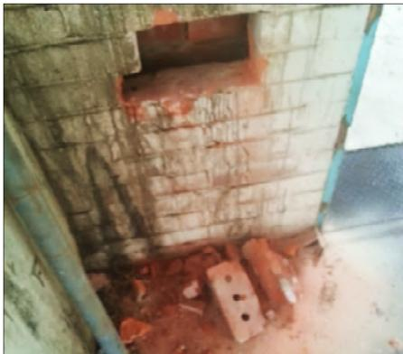
(a) Cavity between two single-brick leaves of hollow-core bricks
