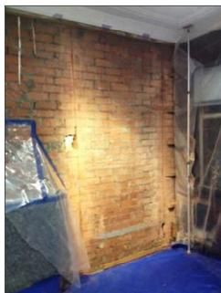
(l) Loaded side of Wel-W6 after gypsum board removal and vertical saw cuts made
