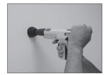
4. Depress the tool firmly against the work surface using both hands, then pull the trigger. Make certain you hold the tool perpendicular to the work. Using the supplied rubber spall stop will help ensure the tool is perpendicular to the work surface and will help to minimize concrete spalling when the fastener is installed.
